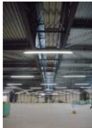
A super-long pillar span of 50 meters makes for great freedom in use of floor space
