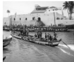
On the job in Ghana
