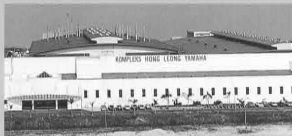
The new 36-acre HLY Complex was opened in 1997, located in St. Buloh, the state of Selangor
