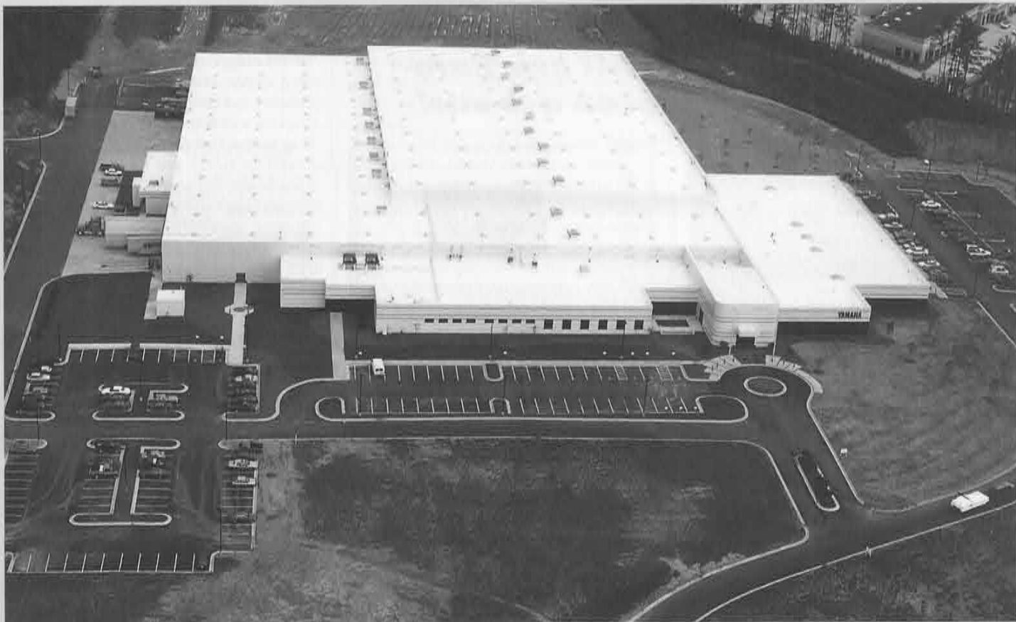
YMUS' new parts center and Southeastern office, located in Kennesaw, Georgia, outside of Atlanta. An 18,000 square meter (194,000 sq. ft.) Parts Center and a 5,500 square meter (60,000 sq. ft.) office and service training center occupy the 37 acre (150,000 square meters) tract
