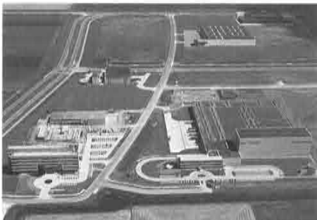
(from front left) European head office, distribution center and service center, currently under construction (completion date December 1993)
