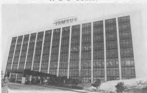
R & D Center which will be completed in the near future, will play the most important part in Yamaha's research & development activities.
