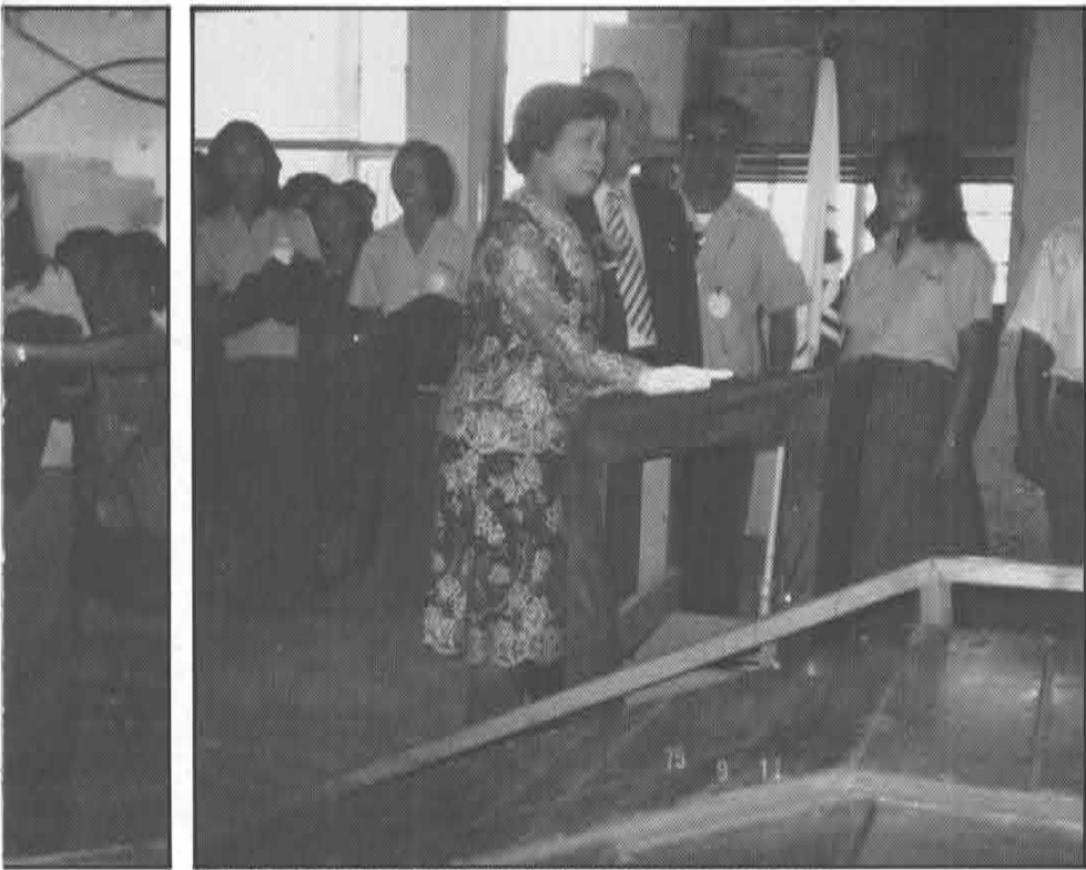
Mrs. Koike pushes the starter button of the conveyor line.
