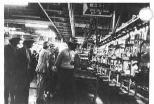
Every work process is smoothly going on
