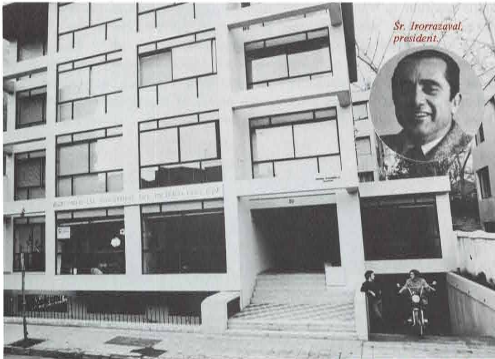
Front view of main office building.
