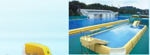
1974 FRP pools created using boat manufacturing technologies
