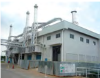
Gas engine generators at YMMWJ [Specifications] Gas engine generators Three generators with maximum output of 2,735kW [Steam used for] resin coating, metal coating, die casting [Reduction of CO 2 emissions by LPG fuel reductions] 400t-CO 2 /year * YMMWJ: PT. Yamaha Motor Manufacturing West Java
