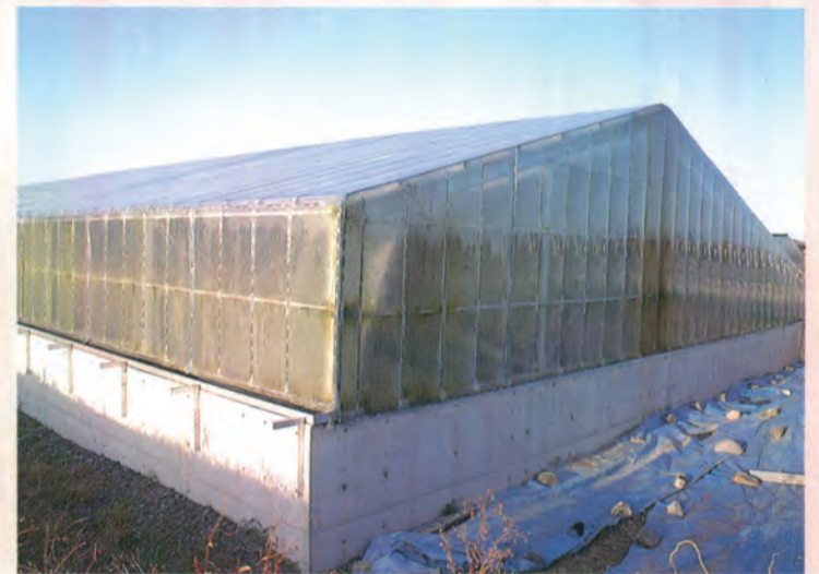
The roof and walls of the hothouse are covered with two layers of vinyl sheeting to maintain the temperature inside.
