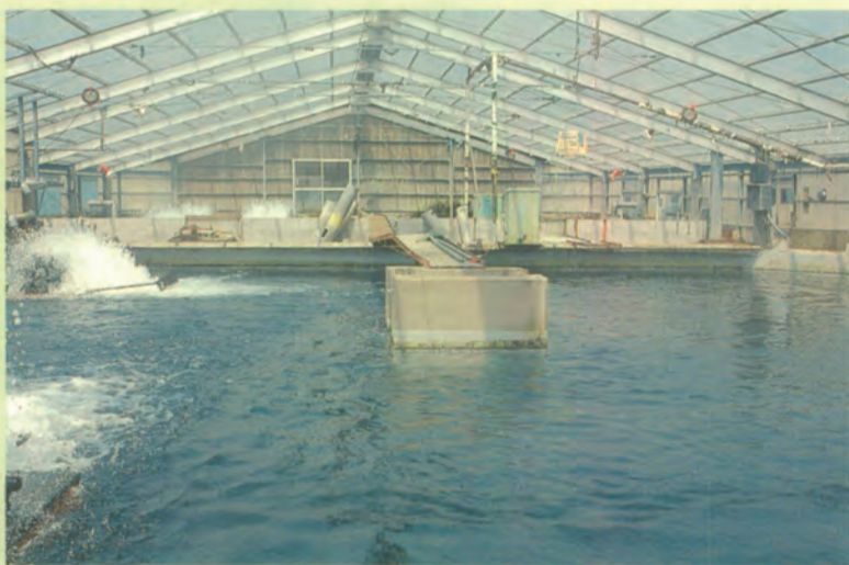
An indoor type culture pond. Indoor type ponds have the advantage of temperature control, but they entail greater construction cost. In Japan, outdoor type ponds are most common.
