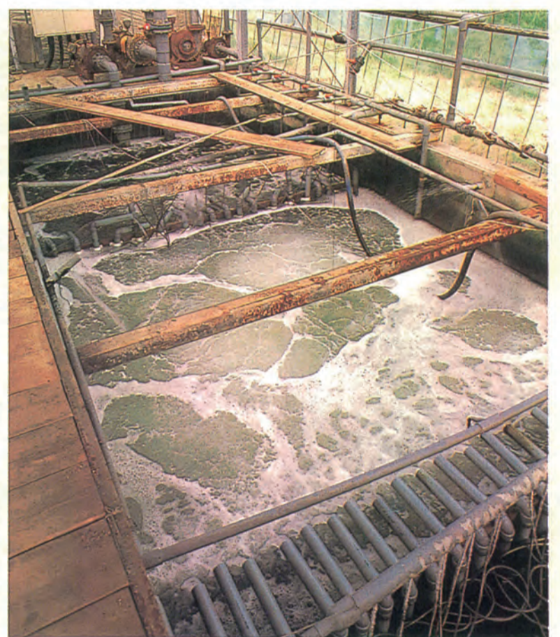
In the circulation/filtration system the water is purified by a combination of physical, chemical and biological means.
