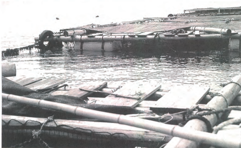
In this area cage frames are constructed of cedar legs with cedar boards tied thereto as strength members and footboards as well.
