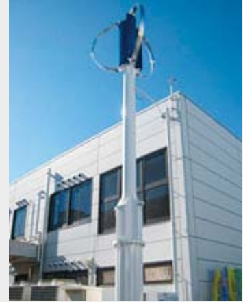
Vertical wind power generation system, which is quieter than the propeller type (Nakaze Factory)
