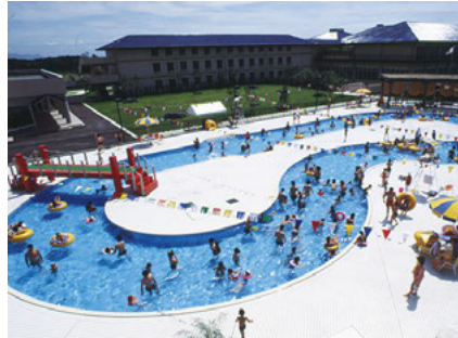
Installed in 1988 (Tsumagoi Water Park)
