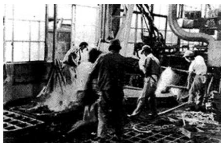
This was the scene of the trials for casting the cylinder, something that heavily influences the engine's performance. The first casting results using the company's piano frame casting technology were laughed at as looking like "teapots." Repeated trial and error and the sweat and tears of the team eventually led to amazingly precise casting capability for the time.
