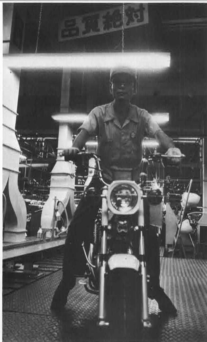
Completion test is one of the most important work processes. Every assembled motorcycle must be thoroughly checked here just before shipment. Four major testing items are sub-divided into 50 points, that's to say, major ones are outlooking, electric equipment, function and cruising. Also, some motorcycles are inspected for power output, fuel consumption, generating, charging, lighting, etc. by sampling method.
