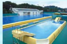
1974 FRP pools created using boat manufacturing technologies
