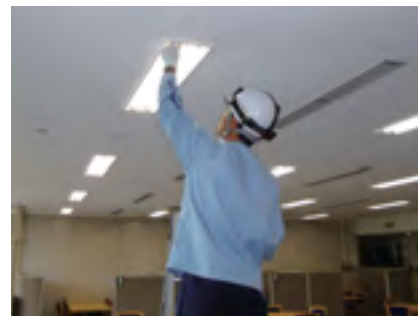
Reducing electricity consumption by replacing from fluorescent light bulbs to LED
