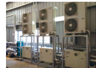
Heat pump at factory in Chennai, India
