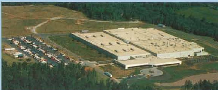
The YMMC building
