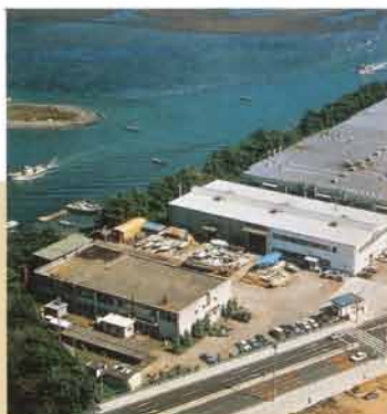
An overall view of the Arai Factory with its 48.628m 2 of grounds and 21,913m 2 of floor space.
