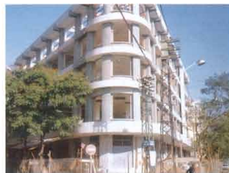
Exterior of the SEAPRODEX office
