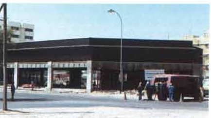
⑥ A new office building nearing completion
