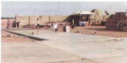
② A new service shop under construction
