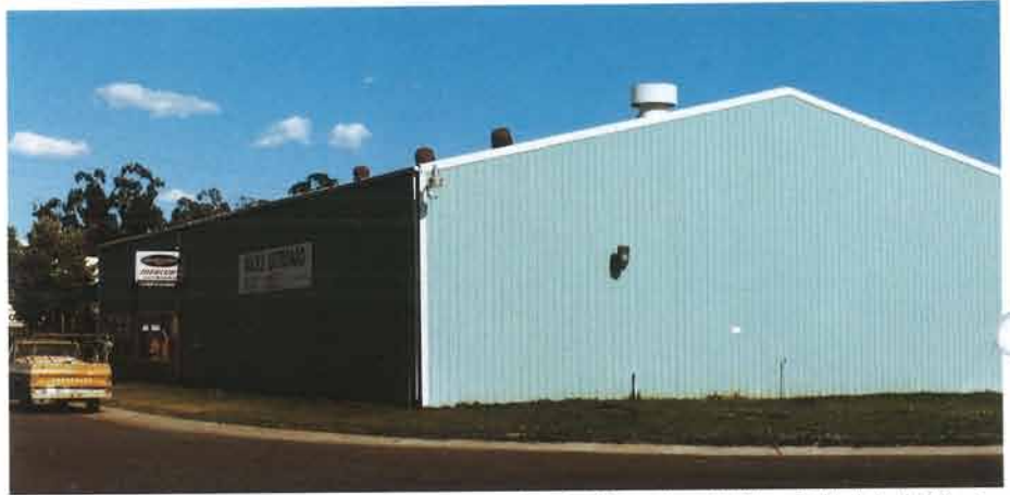
The office, parts storehouse and workshop are all contained in this one large building. Behind the building is a boat storage area.
