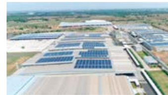
Solar power generation at Chennai Plant (India)
