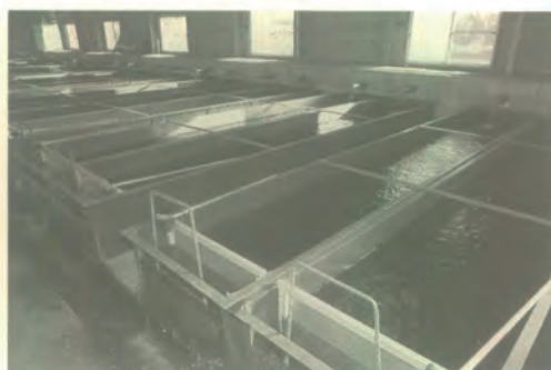
These feeding tanks are made of fiberglass. They are 90cm wide, 6 meters long and 50cm deep (water depth 30cm). One tank holds about 1.6 tons of water. In each tank are kept about 70~80 thousand fry.
