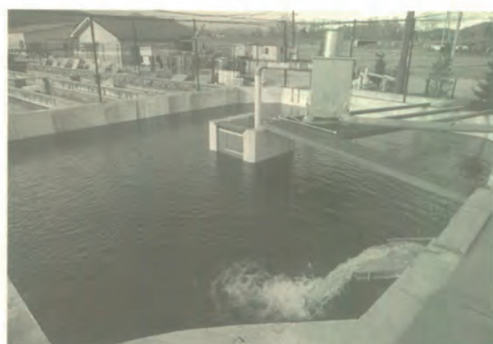
A turtle-shell shaped culture pond. A descending slope extends toward the center where the drain is located.
