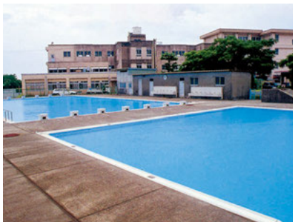
Installed in 1978 (Iwata City Tobu Elementary School, Shizuoka Prefecture)
