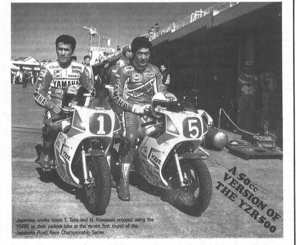
On May 10th an ultra-small sports YSR50 was released on the Japanese domestic market. The new YSR50 is called a tiny replica of the famous YZR500 racer that is seen on road race circuits all around the world today. In spite of the 50cc displacement this bike has a surprising amount of real sports performance and feel. The engine is a highly responsive air-cooled 2-stroke-model.
