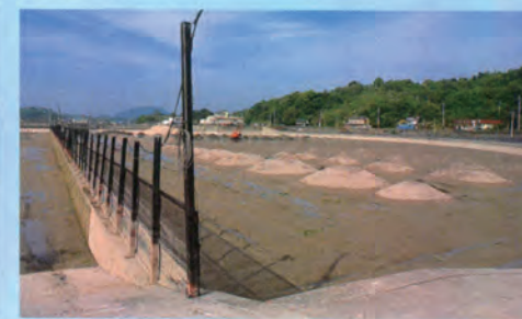
A partial-embankment type grow-out pond that makes use of tidal drop.
