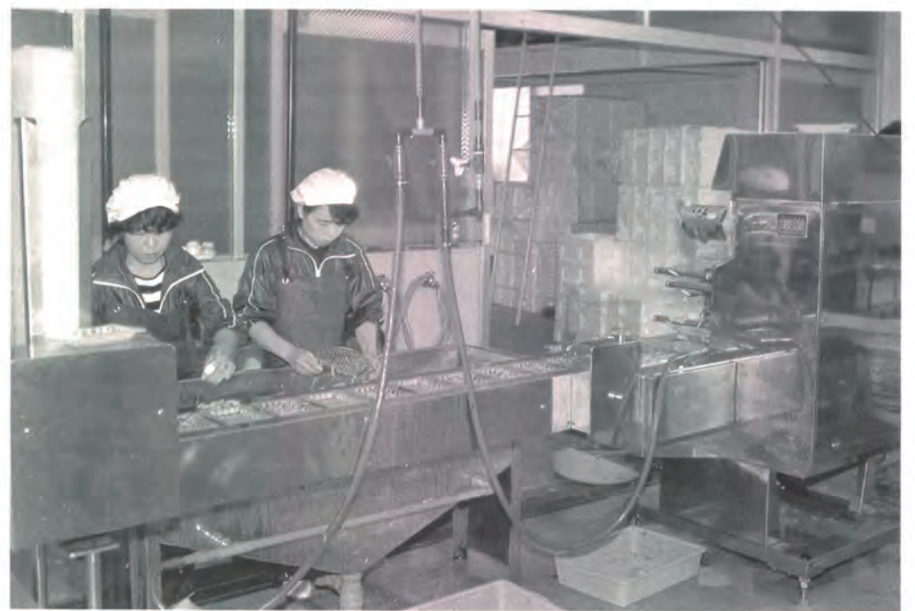
This equipment seals transparent plastic cases automatically.
