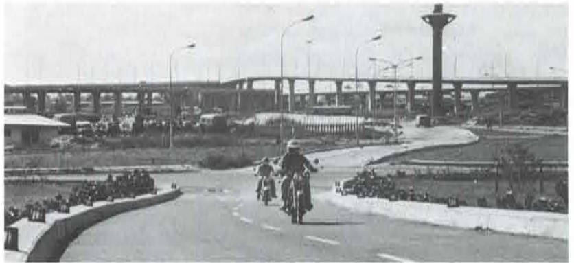
A network of modern highways is being established.
