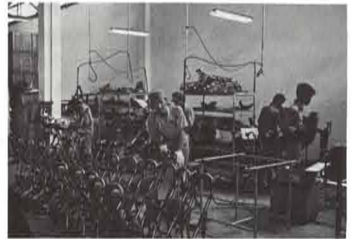
2. Frame welding process
