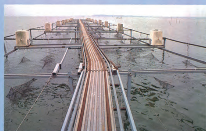
Net cage type culture Net cages are set up along both sides of a walkway extending about 150 meters out from shore. The devices above each cage are automated feeding machines (60kg capacity). The walkway is fitted with a pair of rails for the feed transport car.
