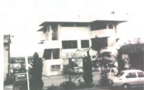
Office building of Uki Fisheries Cooperative
