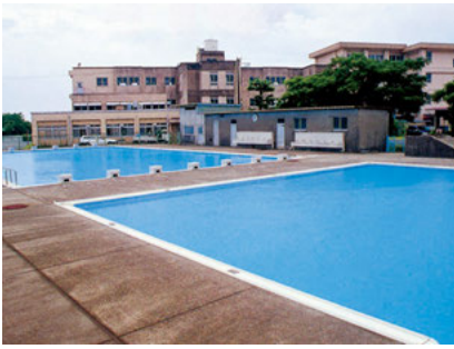
Installed in 1978 (Iwata City Tobu Elementary School, Shizuoka Prefecture)
