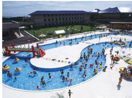
Installed in 1988 (Tsumagoi Water Park)
